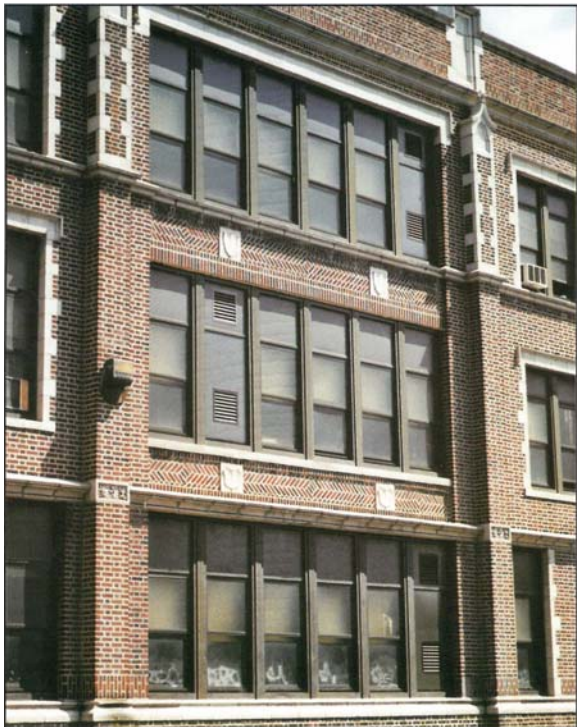
Exterior elevation of a vintage school with vertical unit ventilators louvers.
